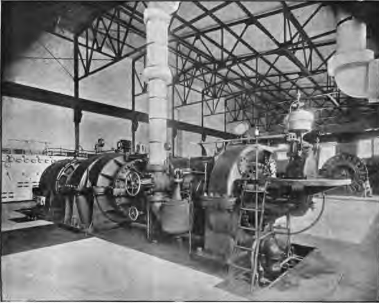
FIG. 9. A 2,000 H.P. WESTINGHOUSE STEAM TURBINE, RESEMBLING THE TURBO-GENERATORS (EACH OF 7,500 H.P.) IN THE CHELSEA POWER HOUSE.
